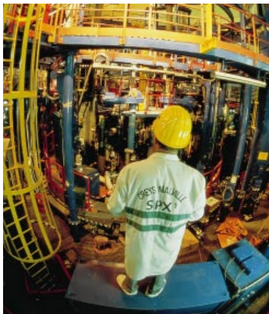
FUEL-HANDLING and coolant-pump machinery are visible in the dome over the Superphénix reactor vessel. The reactor is near Lyons, France.
